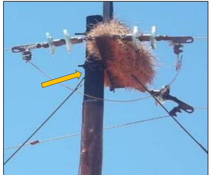
Example of pole-top burn caused by Social Weaver nesting (photo Julia Amukwa).
