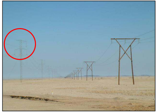
The 66 kV Trekkopje Bypass line (right, with wooden five-pole structures) runs parallel to the larger 220 kV line (left); it is possible that the three flamingos collided with the less visible earth/optic fibre ground wires (red circle above and red arrows below) on the latter structure (photos Ann Scott)
