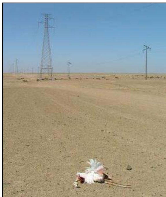
Flamingo mortality on a power line between Swakopmund and Walvis Bay in 2007 (photo Gloudi de Beer)
