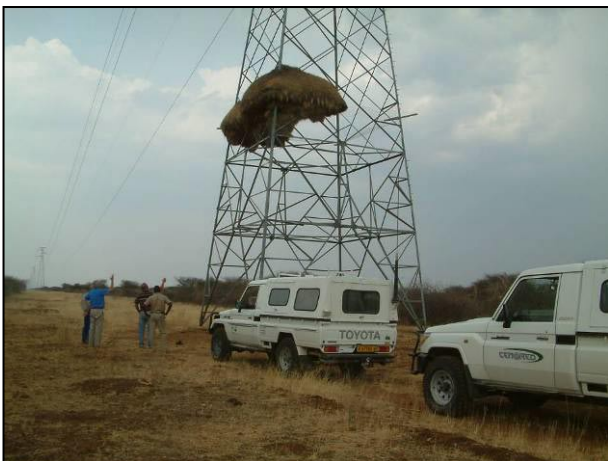
NamPower and Cenored staff accompanied us on a survey of part of the 220 kV Gerus/Otjikoto power line on 24/9/09 (see map above; photo Ann Scott)
