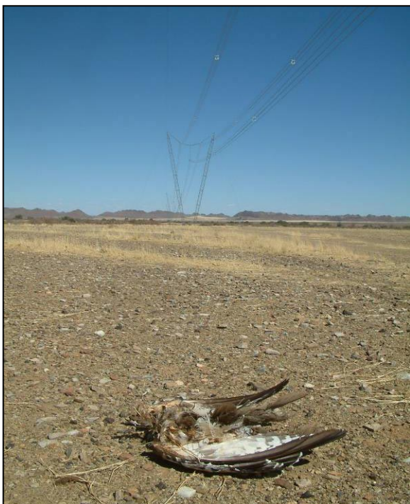
Bustard mortality, apparently due to collision with the near-invisible earth wire of the 400 kV Kokerboom line east of Keetmanshoop - see p2 (photo Ann Scott)
