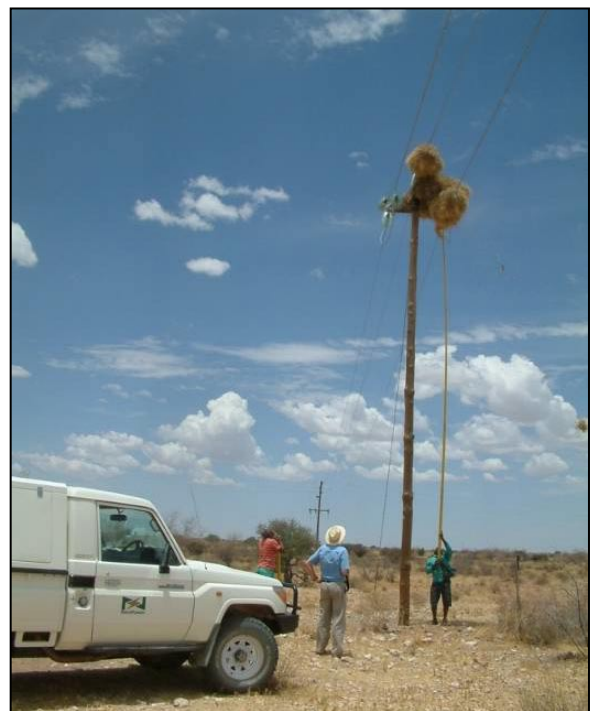
Removal of Sociable Weaver nests that cause outages on the 33 kV HLPD lines east of Mariental, especially during the rainy season – see p3 (photo Ann Scott)
