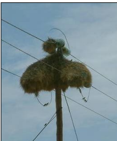
Sociable Weaver nests on HLPD lines (left) cause outages, and the poles may catch fire (centre and right; photos Ann Scott)
