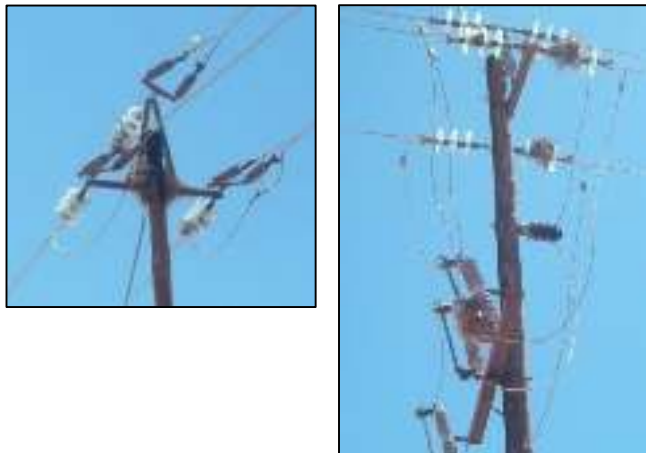
Figure 2 (left). Burnt pole with two birds actively nesting Figure 3 (right). Multiple nests of one pole.
